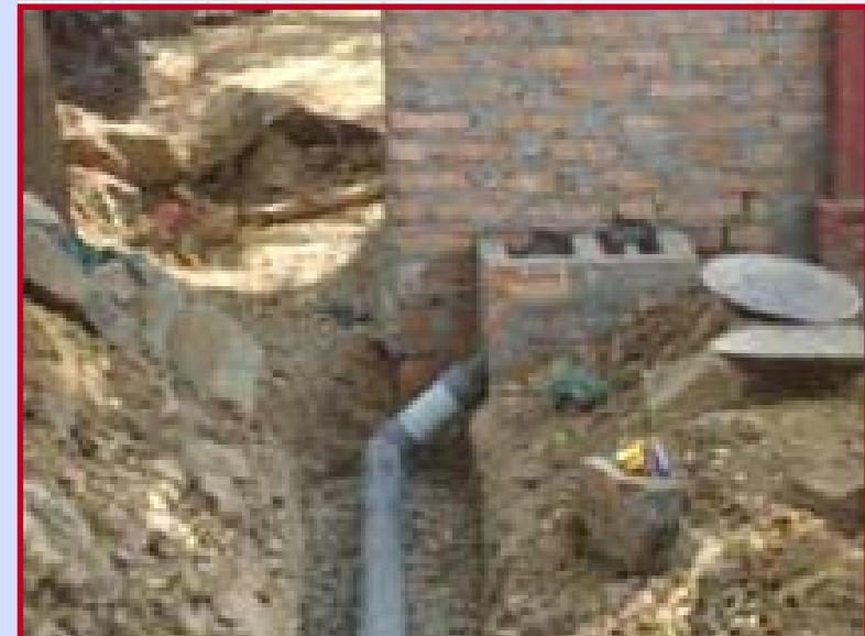
the twin pits. This kind of construction implies infiltrations pipes made from normal pipes which have been partially cut with 5 mm slits, concrete boxes (inlet and outlet), a plastic sheet and geo-textile brought from France to prevent entrance of soil in the filter.
